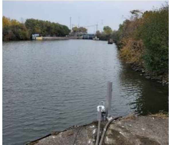
USGS streamgage 05538020, Des Plaines River, Illinois near the Brandon Road Lock and Dam Source: USACE
