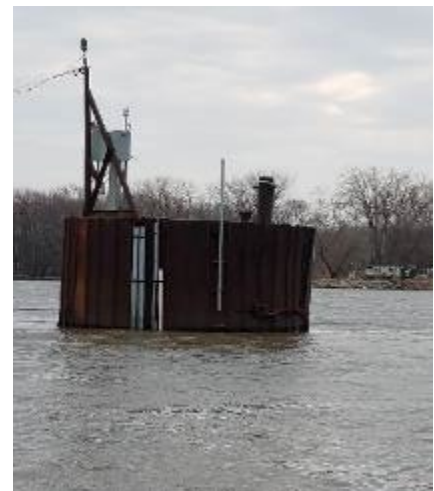
Photograph of USGS real-time, continuous water quality monitoring station 05543010 on the Illinois River at Seneca, Illinois. Photo credit: USGS
