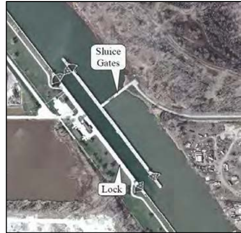
Figure 12. Sluice gates at Thomas J. O'Brien Lock and Dam.
