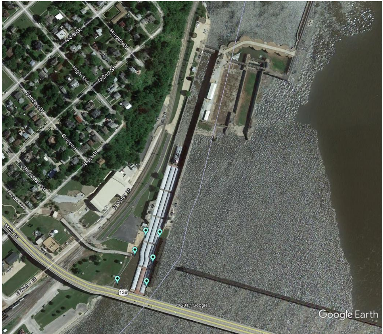
Figure 5. Location of receivers to be installed at Lock 19.
