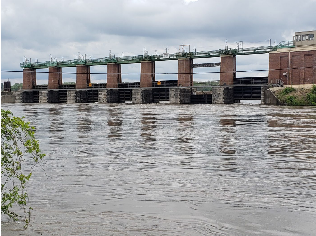
Photo 1. Picture of Bear Trap Dam Control Works. Picture was taken May 18, 2020 from the entrance of the low water crossing to get to Cargill Boat Ramp looking East-Northeast. Water levels appear to be very similar between the water bodies.
