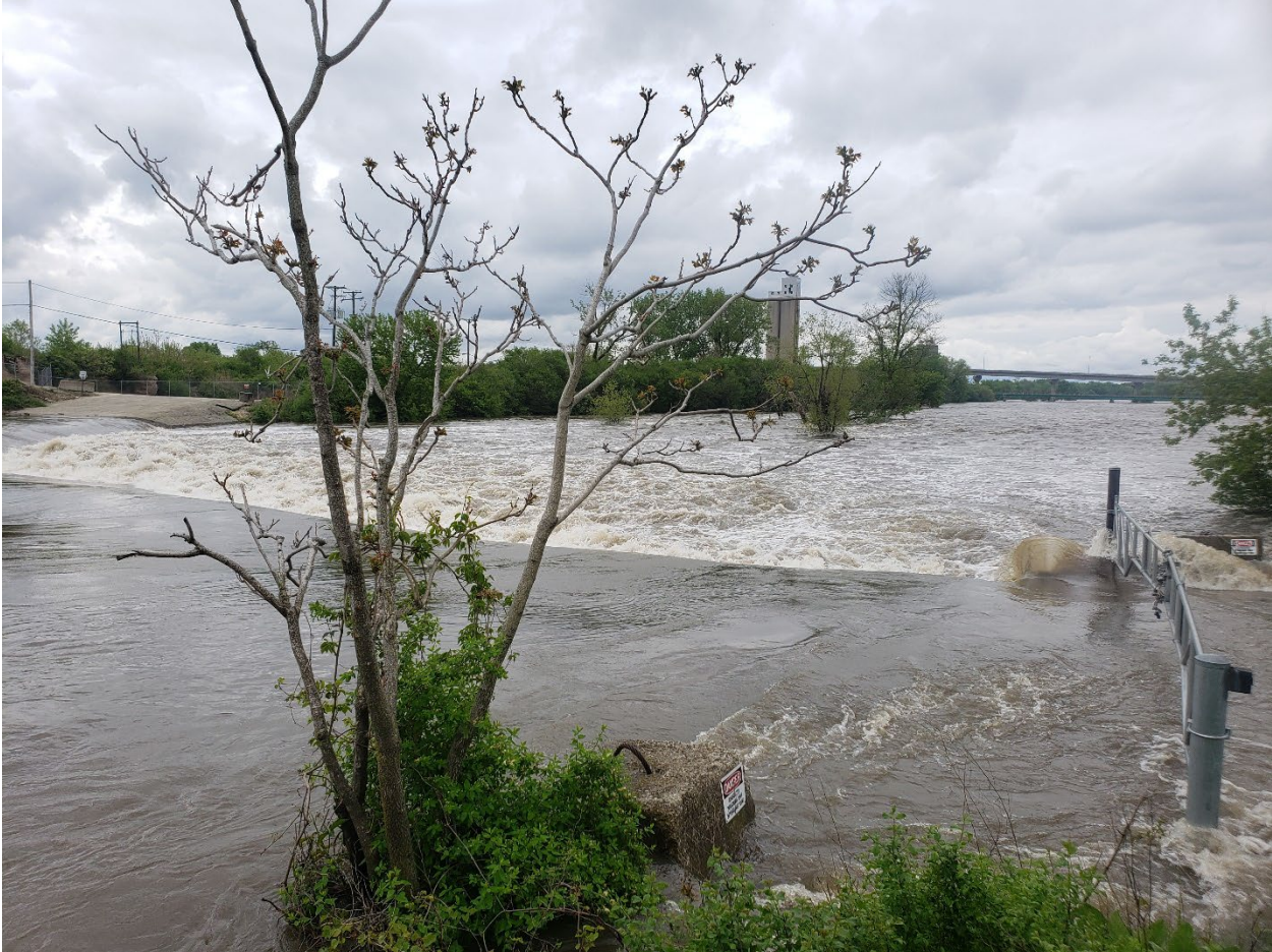
Photo 2. Picture of water flowing over the low water crossing road on the way to the Cargill boat ramp. The picture was taken May 18th, 2020 looking south-southeast.
