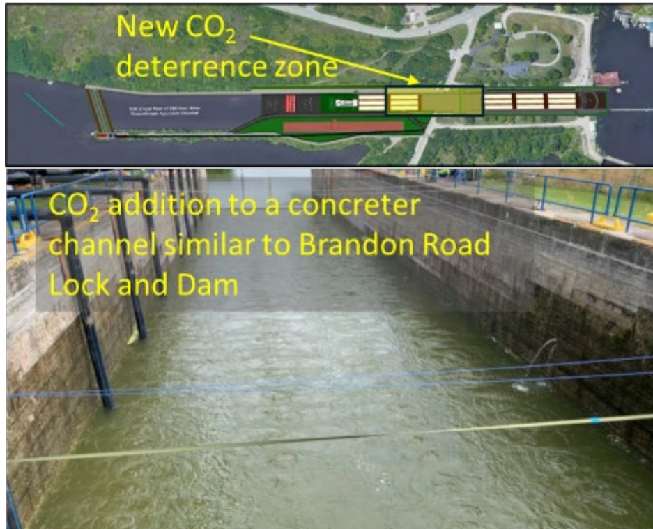
Figure 11 — Carbon Dioxide Deterrence Zone at BRIP
