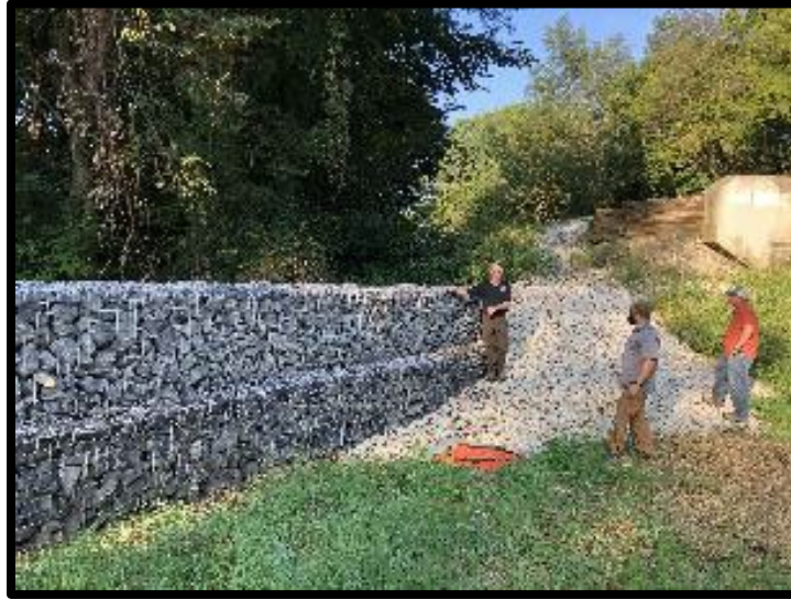
Photo of the Gabion Basket Barrier at the Ohio & Erie Canal. Source: OHDNR
