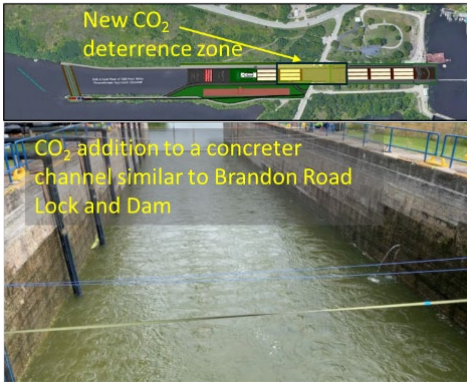
Figure 10 – Carbon Dioxide Deterrence Zone at BRIP
