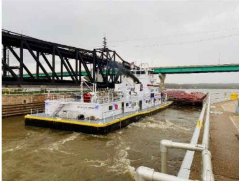
A downbound tow and barges traversing downstream lock approach channel over the UADS at Lock No. 19. Photo credit: Christa Woodley, USACE ERDC
